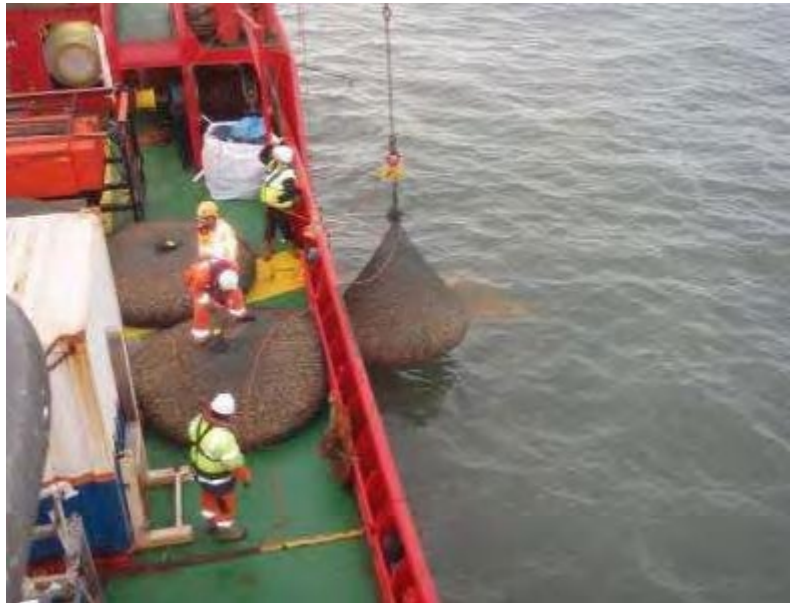
Plate 4-15: Rock bag installation (Source: Equinor)
